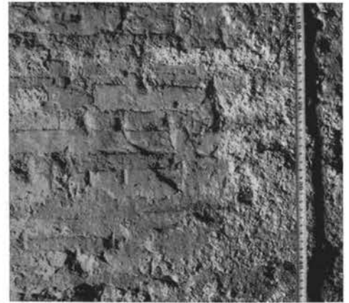
Fig. 89c. S. Martino ai Monti, Roman Hall, brickwork a, third century
